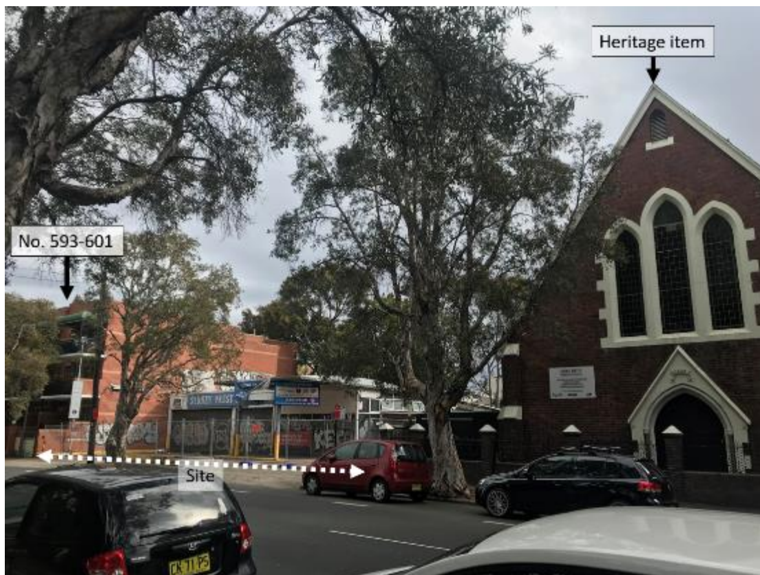
Figure 3: Looking south-west from Elizabeth Street
