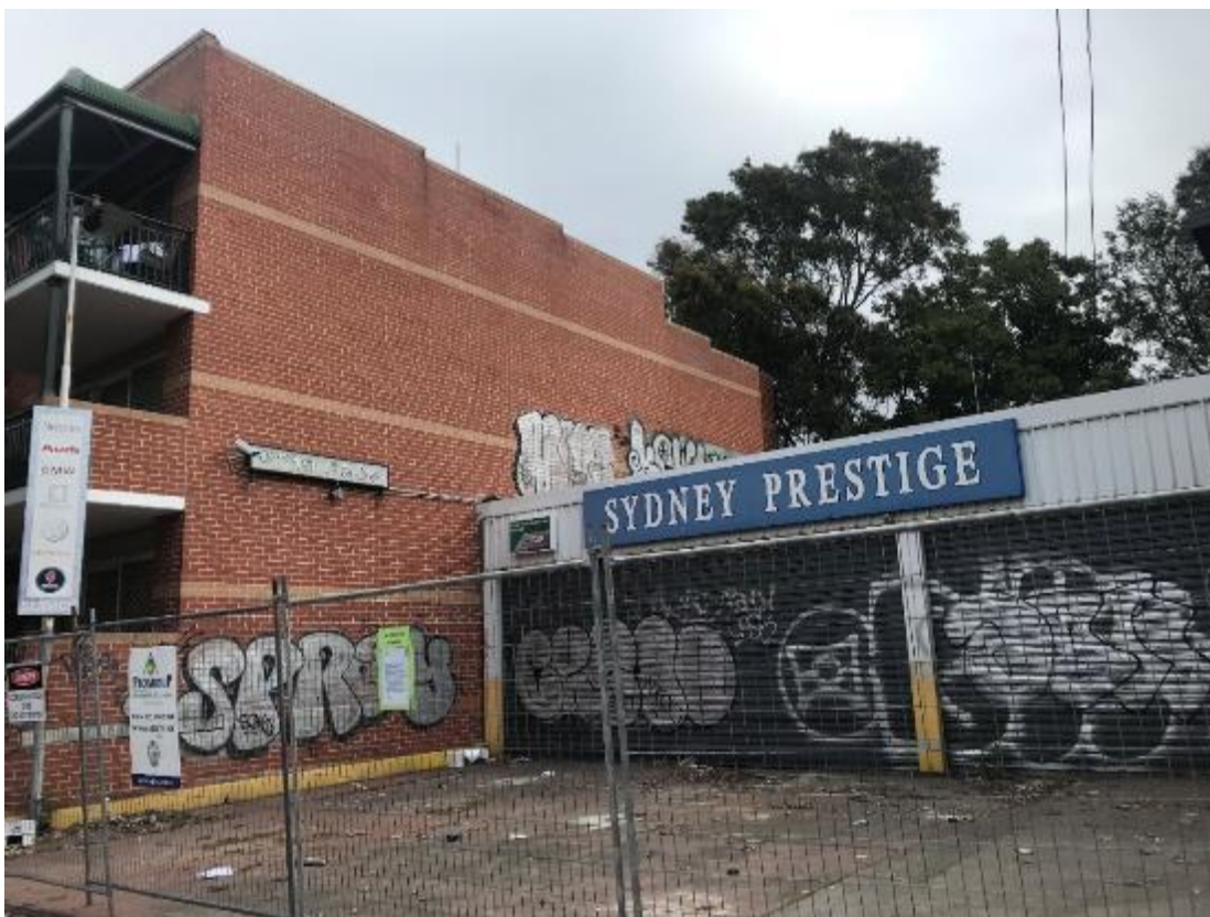
Figure 9: View from Elizabeth St of site and adjoining residential flat building at 593-601 Elizabeth St
